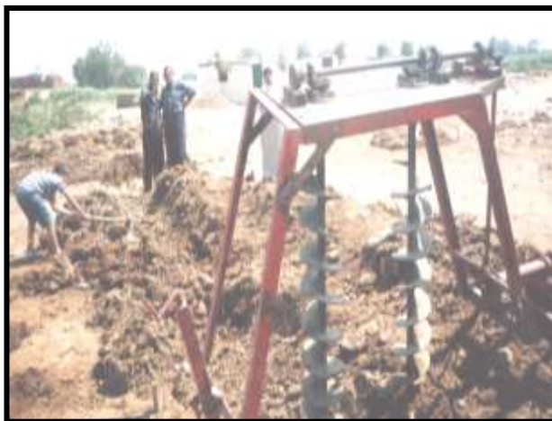
Fig. 6 : Upright turning machine during work on long pile .
