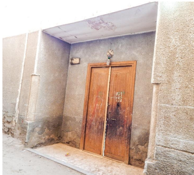
(Fig. 9) The outer northern entrance to the church. (The researcher)
