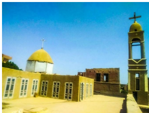
(Fig. 36) The Roof of the Church. (The researcher)
