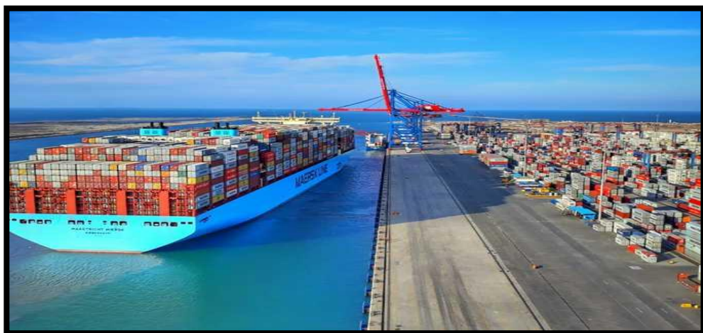
Figure (1): East Port Said Port.
