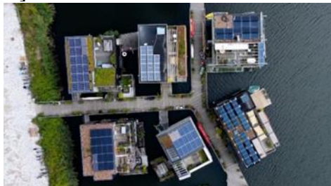
figure 12 roof-top solar collectors [9]
