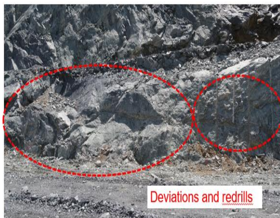
Figure 12 Borehole deviation and redrills.
