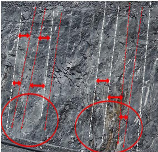
Figure 11 Common presplit drilling errors.
