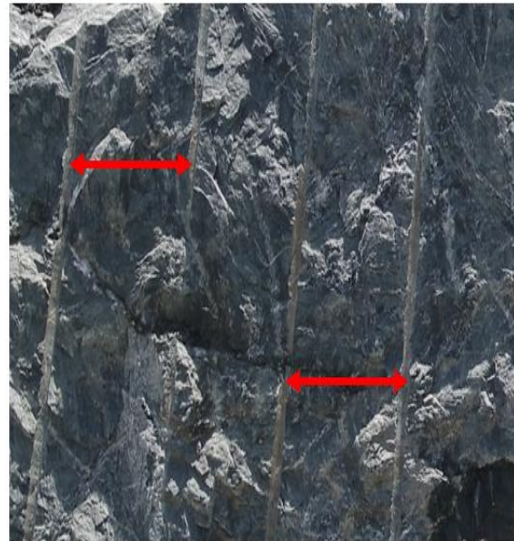
Figure 13 Improved presplit drilling and blasting.
