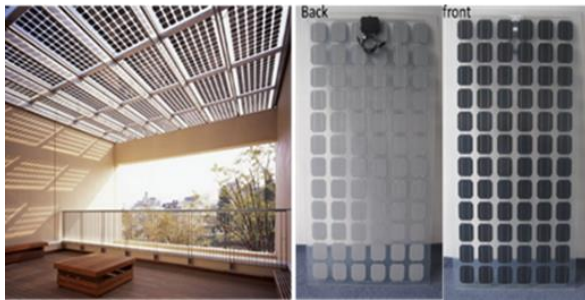
Fig. 5. Examples of transparent crystalline panels used as skylight
