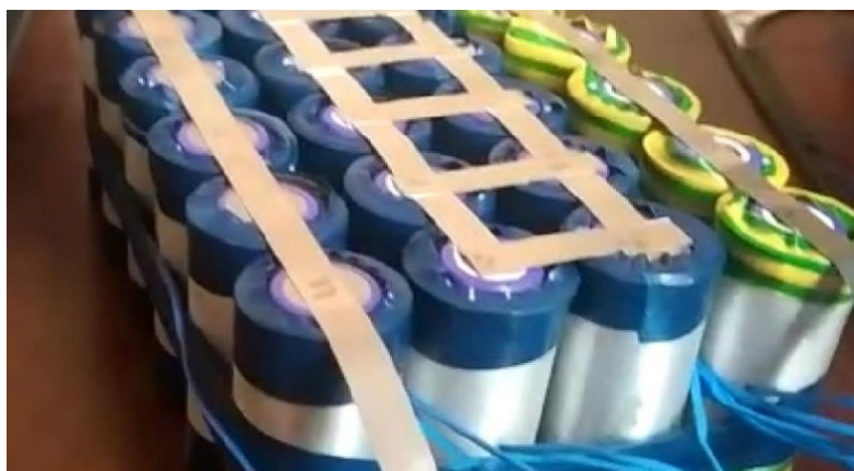
Fig.5 Batteries and phase change materials unit
