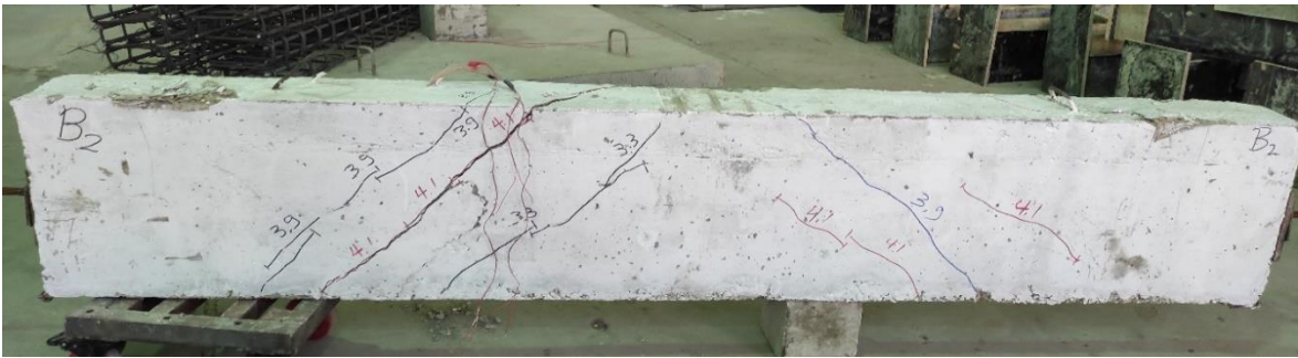
Fig. 7. Crack patterns at failure of specimen (B2).
