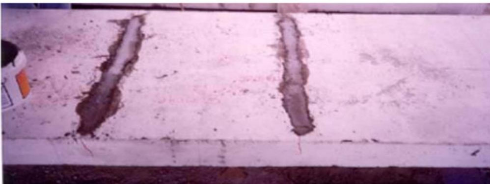
Fig. 3: using the grout pouring technique to mend cracks [18]
