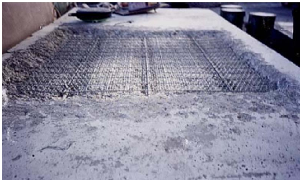
Fig. 5: Wired mesh used for repair [18]
