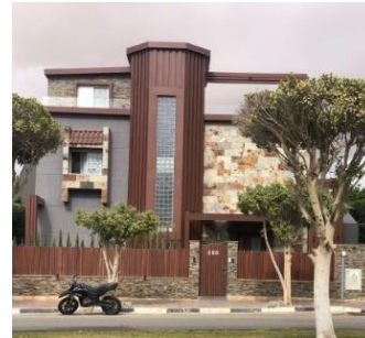
Figure 20 Personal Status is shown when one owner decides to change the whole façade with different materials and colors. Authors, 2024
