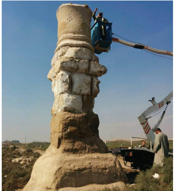
During work at the Beni Hasan site.
