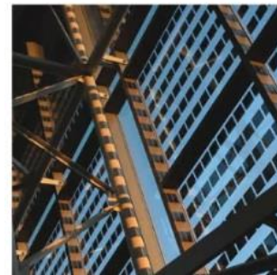
Fig.9 Glass curtain wall with integrated photovoltaic. Source: (Green Studio, 2024).
