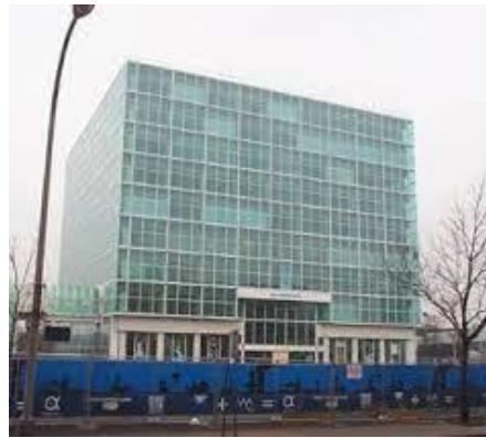
Fig. 8. shows the Occidental Chemical Center– Niagara Falls using the double casing system in the facades.
