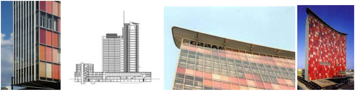
Fig.12. shows GSW Company and Shadows on the west façade created a thermal buffer zone between the inside and the outside and the shape of the parachute above the tower.
