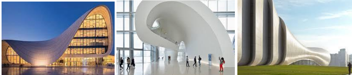
Fig. 16. shows reinforced concrete with glass fiber in the interfaces of the Hyder Aliyev Center
