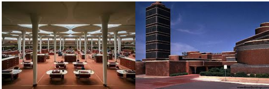
Fig. 3. shows Johnson's wax company building and shows the lab tower as well as the main lounge showing the cone columns.
