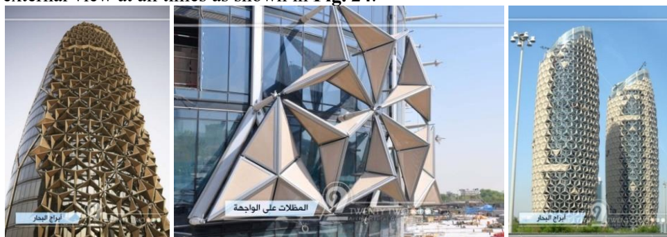
Fig. 24.shows Sea Tower Abu Dhabi
