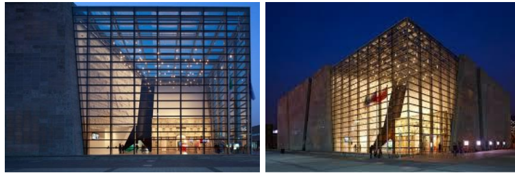
Fig. 15. shows the Use of transparent concrete in Italian wing facade in Italian Pavilion in Shanghai
