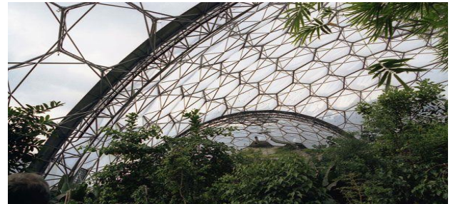
Fig 12. Iron Structural Meshes of Eden Project, Saint Austell (Cornwall) [24].
