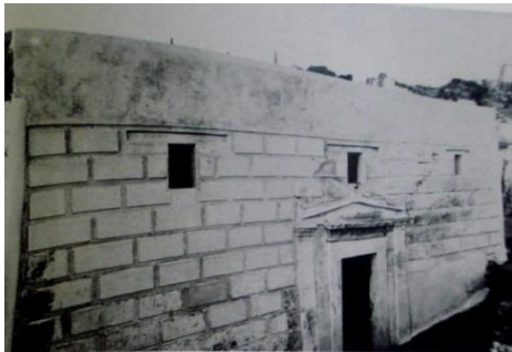
Figure 18: the facade of House Tomb 21 , Tuna El-Gebel combines the Egyptian cavetto cornice and a triangular Greek pediment (after Riggs, 2005,131)
