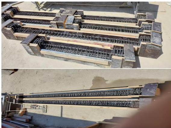
Fig 2: Columns Formwork and Reinforcement Cages
