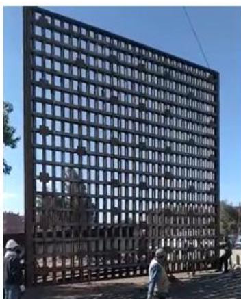
FIGURE 4. Bridge sleepers in an upright position raised for repair
