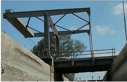
FIGURE 2. General view of the steel bridge before rehabilitation
