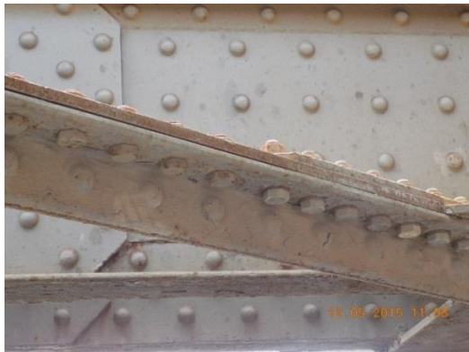
Fig.(13) rivet and bolt in one connection – Edfina bridge
