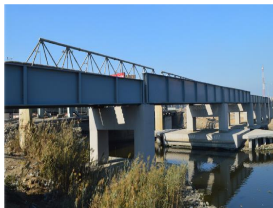
Fig.(2) Raswa Bridge, Benha - Port Said Line, 1987
