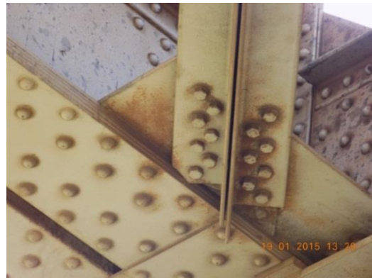
Fig.(14) Replacement of rivets with bolt – Kanater bridge
