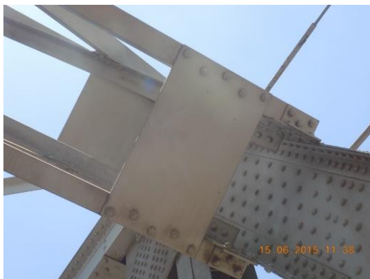
Fig.(11) Replacement of rivets with bolt – Dessouk bridge
