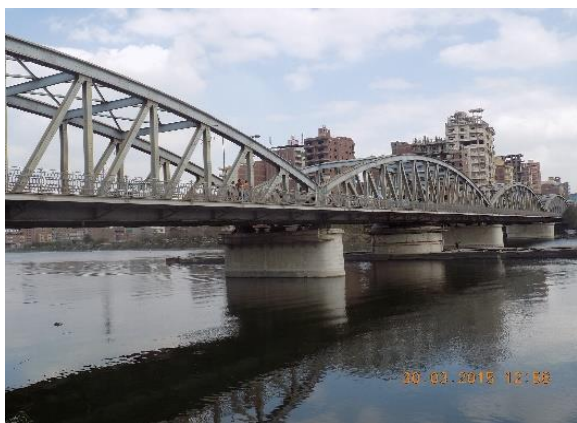
Fig.(1) Zefta Bridge, Zagazig - Zefta - Tanta Line, 1907
