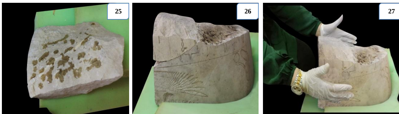
Fig (25-27) shows The application of epoxy on a small stone piece in preparation for bonding it and completing the attachment of the two stone pieces.
