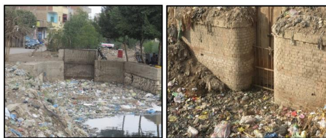
Fig. 3. Debris accumulation upstream covered channel.
