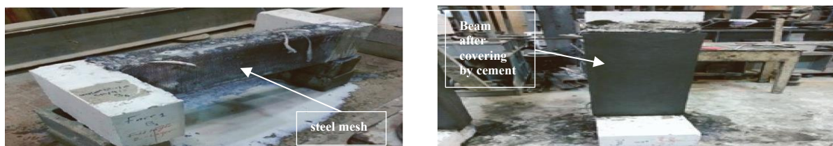
Figure 12. Details of the repair techniques.[10]
