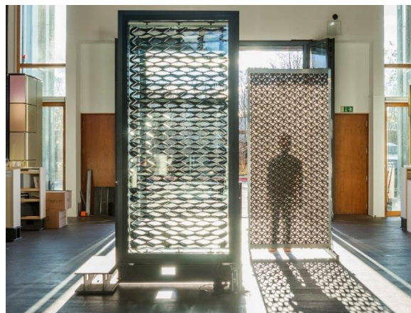
Figure (5) Adaptive facades act as smart materials (shape memory alloys) as a shading solution [10].
