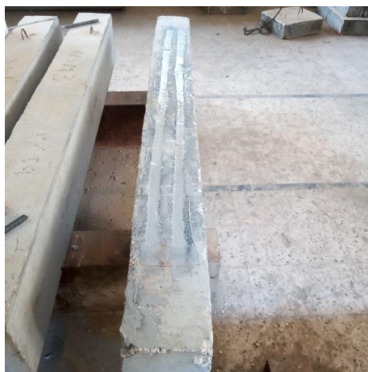
Fig. 6 Beams after the installation of the NSM bars.
