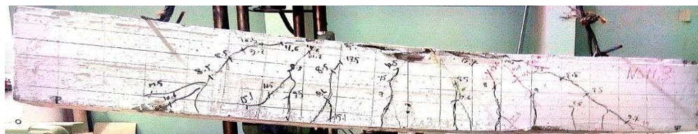
b) Crack pattern and mode of failure for beam (NSM3).
