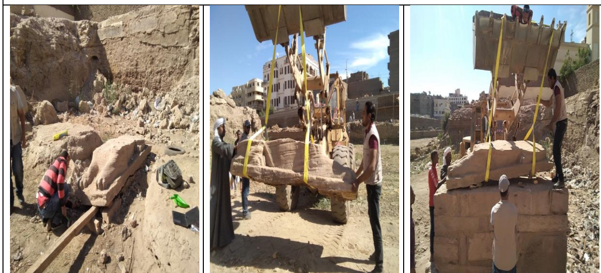
Figure 15. Shows the process of raising and fixing one of the statues' bodies on the base after reconstruction processes.
