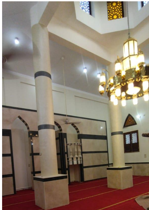
Figure 5; Marble reinforcement of walls after reinforcement and insulation operations with raising the level of the foundations.
