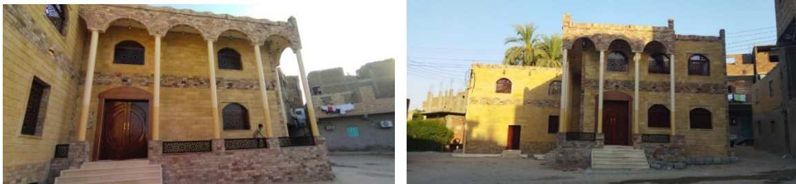
Figures 4. A, B raised from the ground by about 120 cm, with reinforced with stones.
