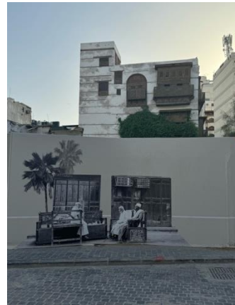
Figure 4: Construction site covered with interpretive design.
