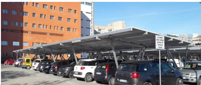
Figure 5: Applications of photovoltaic systems for covering parking-[24]
