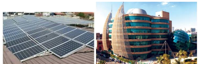
Figure 11: Solar panels at 57357 Hospital-[37]
