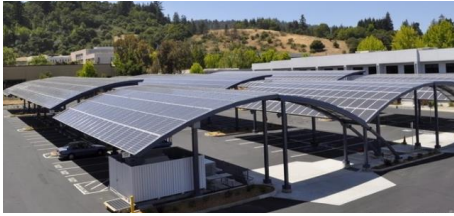
Figure 8: Installation of solar cells on curved roofs- [31]
