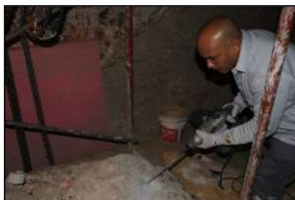
Fig (22) Using the drill device to make accesses for stainless steel bars
