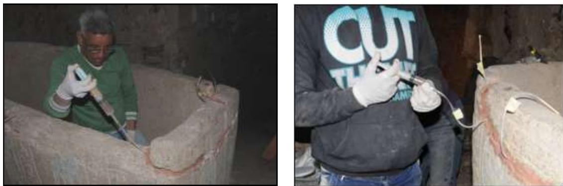
Fig (20) Cracks grouting using Araldite 1092 with fixed injection hoses
