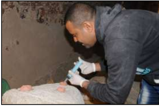
Fig (23) Araldite 1092 injection by syringes
