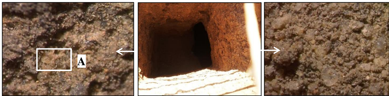
Fig. (14). the infrastructure soil of Ramses II pylon and the samples on which tests and were conducted.
