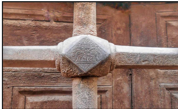
Fig. (2): shows one of the metal grilles in the mosque of Prince Qajmas Al-Ishaqi, and the rank of Prince Qajmas Al-Ishaqi appears on it after the surface layers that were hiding it were removed by mechanical cleaning.
