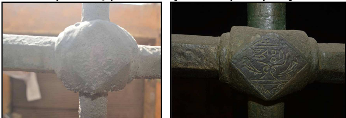
Fig. (14): Shows the blazon of Prince Qajmas Al-Ishaqi on the surfaces of the grilles before and after treatment and conservation processes.
