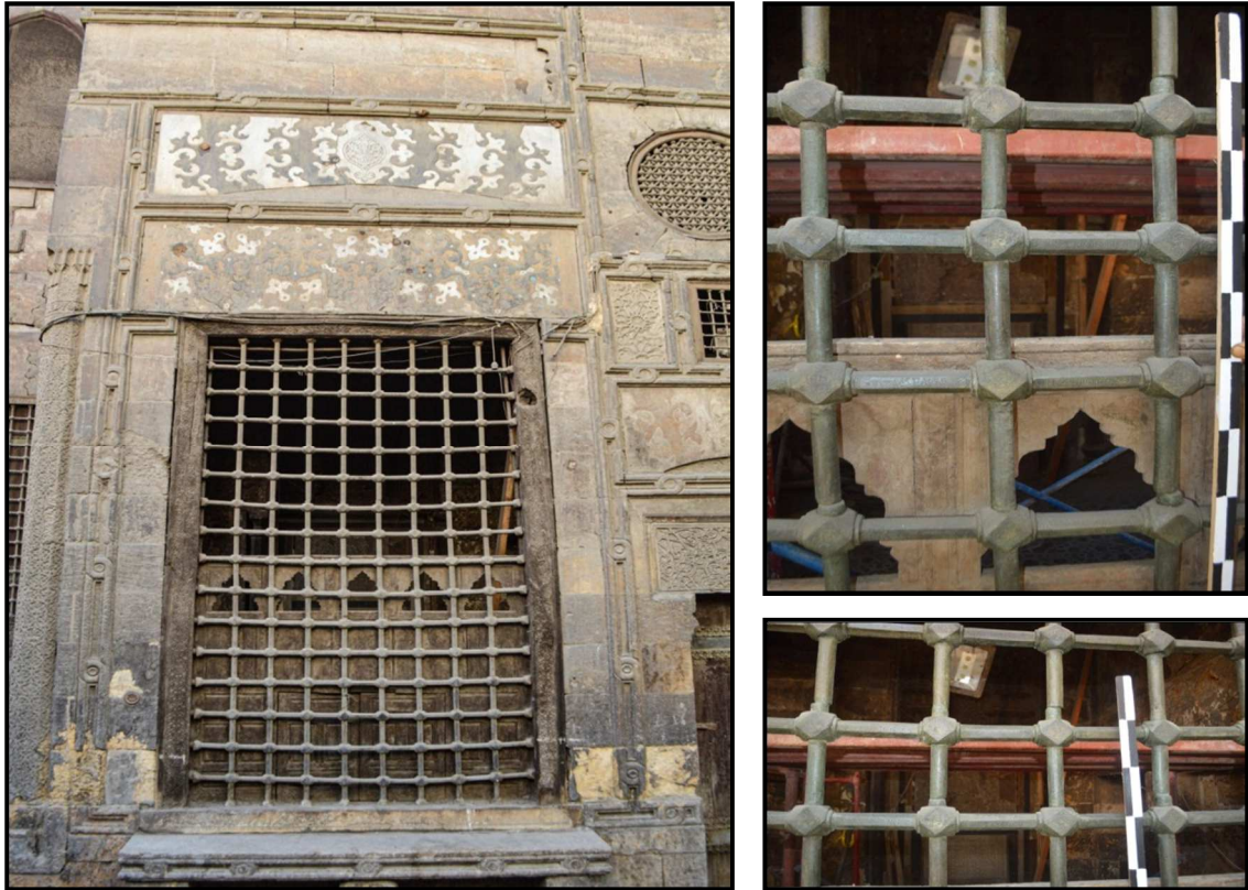
Fig. (13): Shows the grilles of the Sabil window of the Prince Qajmas Al-Ishaqi Mosque after the treatment and conservation processes, and displaying the blazon of Prince Qajmas Al-Ishaqi on the surfaces of the grilles.
