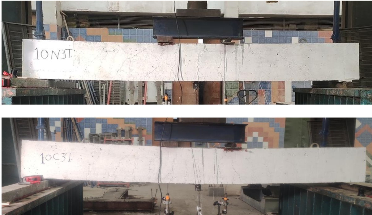
Figure. No. 5: Cracks of Specimens 10N3T and 10C3T at serviceability loading stage
