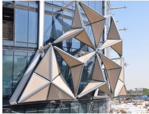
Fig. 4. Various positions of the external triangular units according to the external environmental conditions provide flexibility with all conditions [30].
