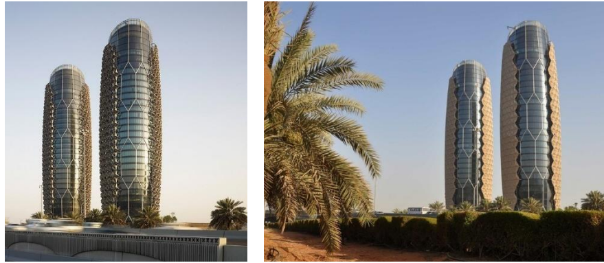
Fig. 1. The external architectural composition of the twin towers of the Abu Dhabi Sea Towers and their relationship with the surrounding local environment. On the right is the complete closure of the triangle units, and on the left is the opening of those units during daylight hours [29].
