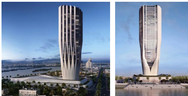
Fig. 6. The distinctive architectural design of the northern facade on the right and the southern facade on the left of the Central Bank of Iraq building [31].
