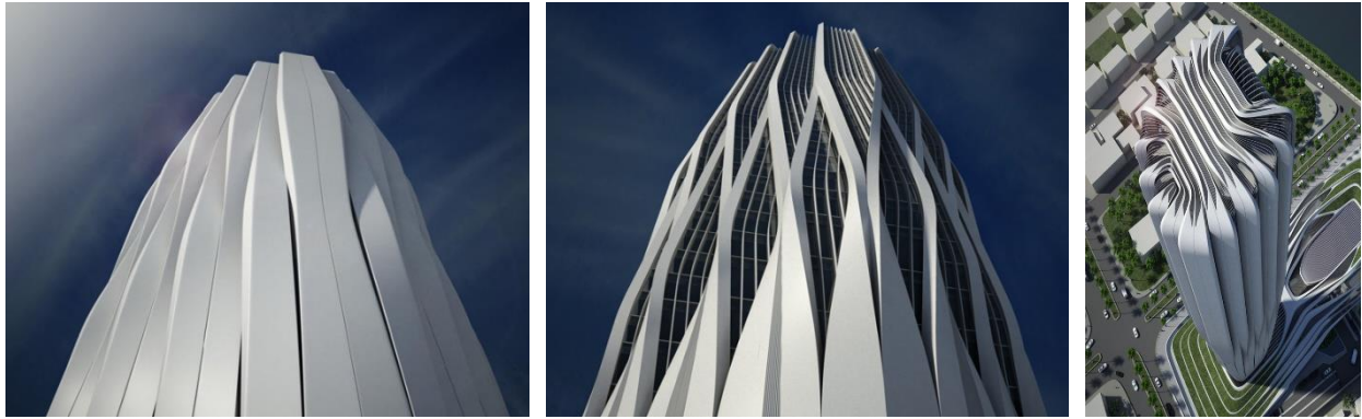
Fig. 7. The dynamic design of the sun breakers changes with height along the body of the building as the angles of sunlight change to the facades of the Central Bank of Iraq building [31].
