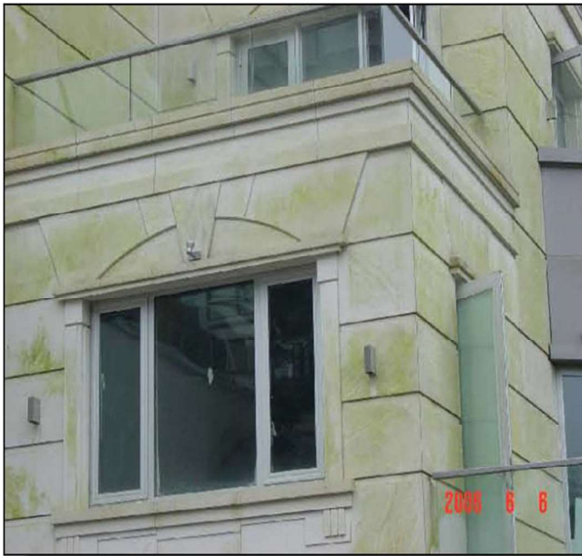
Fig.2. This picture shows a granite wall which has become old and dirty after years of weathering
