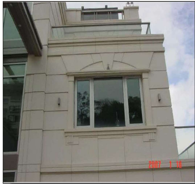
Fig.2. This picture shows a granite wall which has become old and dirty after years of weathering
