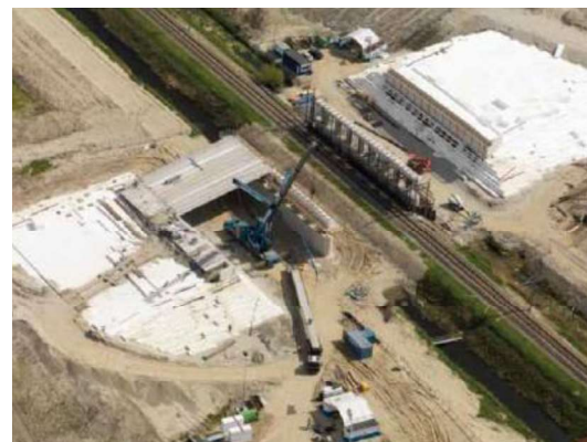
Fig 10 rail embarkmet with geofome USA
