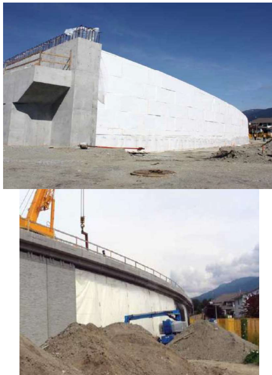
Fig 7 St. Louis, Missouri under an active bridge along Tucker Boulevard, USA
