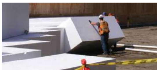
Fig 4 Alaska Way Viaduct in Seattle, Washington, USA
