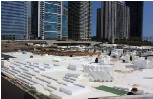
Fig 11 geofome in the construction phase in millennium park Chicago, USA.
