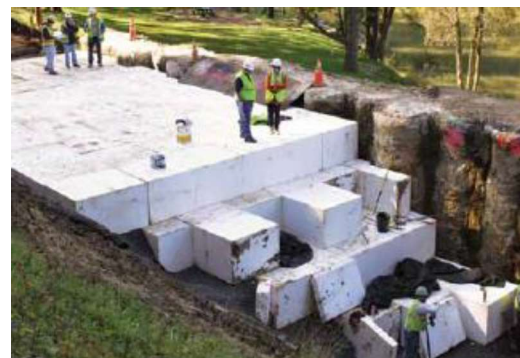
Fig 13 Repair unstable slopes along County Highway Duncan, British Columbia, Canada
