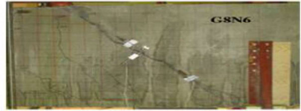
b. Exp. Crack Pattern for (G8N6)
