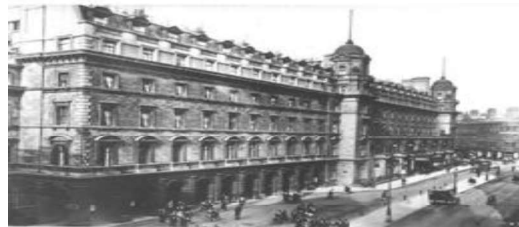
Figure 15: The old Birmingham New Street. Source: https://en.wikipedia.org
