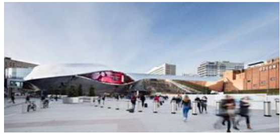
Figure 14: Birmingham New Street Station, UK. Source: Mairs, J. (2016).
