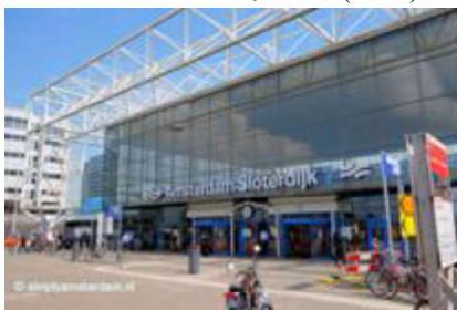
Figure 12: Sloterdijk Station, Netherland; by H. Reijnders of, Holland Railconsul. Source: http://www.simplyamsterdam.nl
