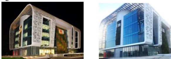
Fig. 1 The Current Situation of CIB After Building Envelope Retrofitting.
