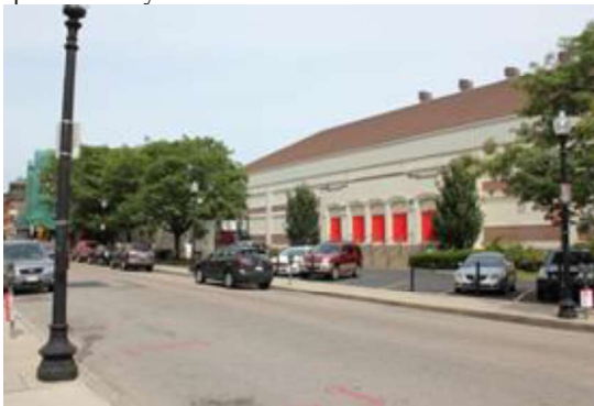
fig. 11: A picture shows the changes made in the library's facade
