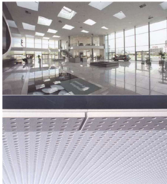
Figure 3: Air Purifying material in an office building, (Leydecker, 2008)
