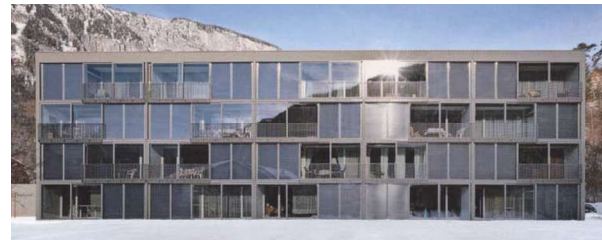
Figure 8: "Sur Falveng" housing for elderly people exterior shot, Zurich, Switzerland, (Elvin, 2007)
