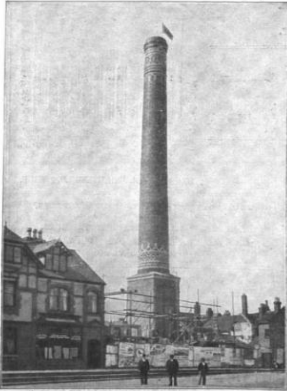
Chimney Shaft, Corporation Electricity Works, Worcester. 150 ft. x 7 ft. 6 in.
