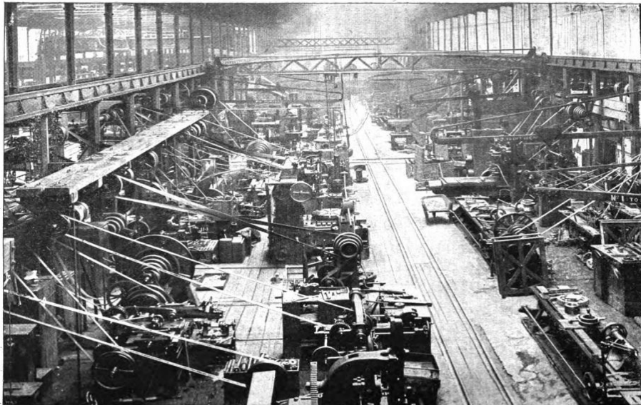
MACHINE SHOP, Messrs. EASTON, ANDERSON & GOLDEN, LIMITED, EATH IRONWORKS.
