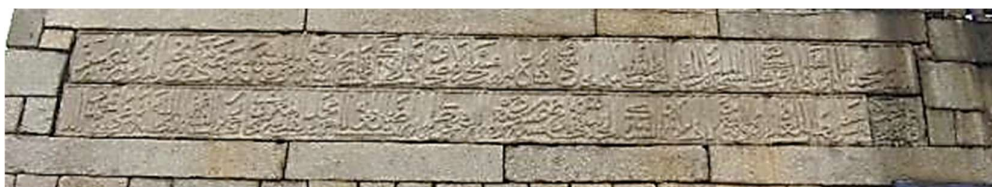
Fig. 5 The construction inscription 710 AH/ 1310-1311 AD
