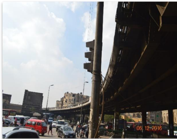
Figure 1: General View Of Curved Part Bridge
