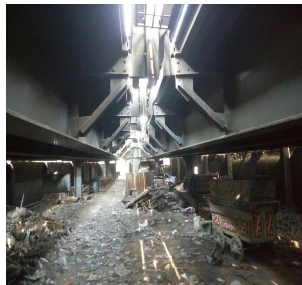
Figure 18: Adding Bottom Steel Plates To Increase Stiffness Of Supporting Beams And Diagonal Bracing To Cross Beams
