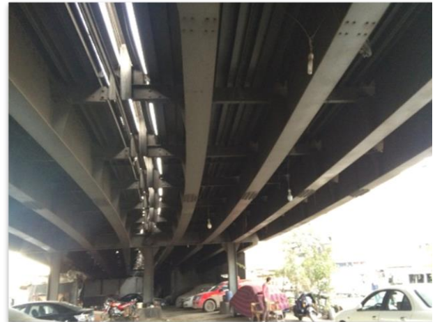
Figure 2: Main Beams Of Bridge
