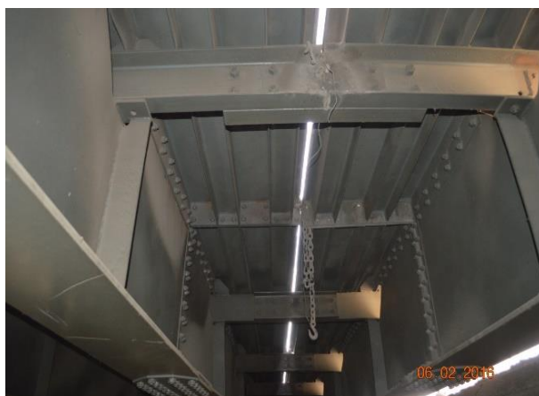
Figure 3: Orthotropic Deck System
