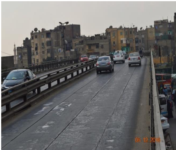
Figure 11: Lack Of Speed Limit Signs
