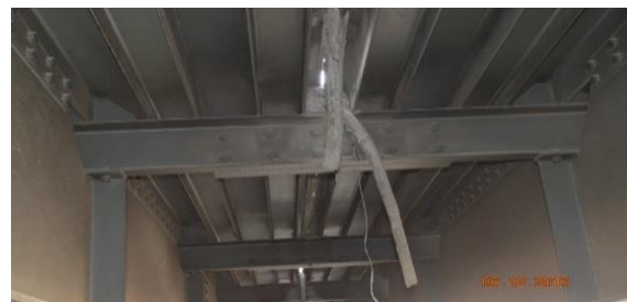
Figure 15: Relation Between Cross Beams And Metallic Deck
