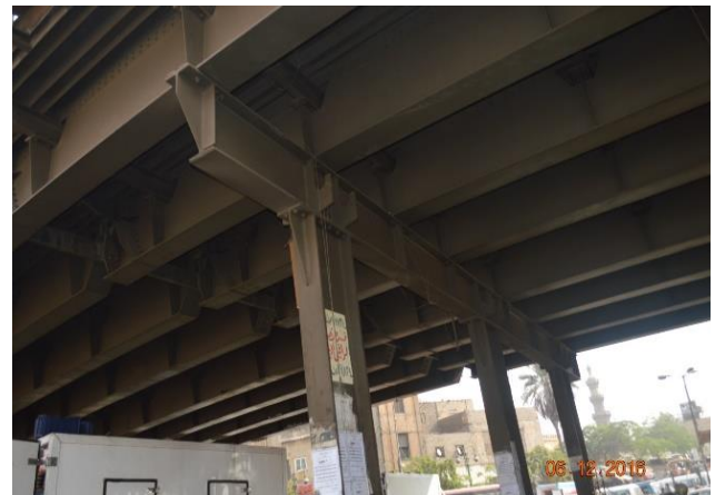
Figure 4: Supporting Steel Moment Resisting Frame
