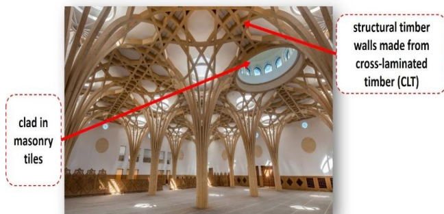
Figure 12 Prayer Hall structure features digitally fabricated tree timber columns supporting the roof structure. Source: “ https://www.dezeen.com/2021/01/20/cambridge-central-mosque-marks-barfield-architects/ .”
