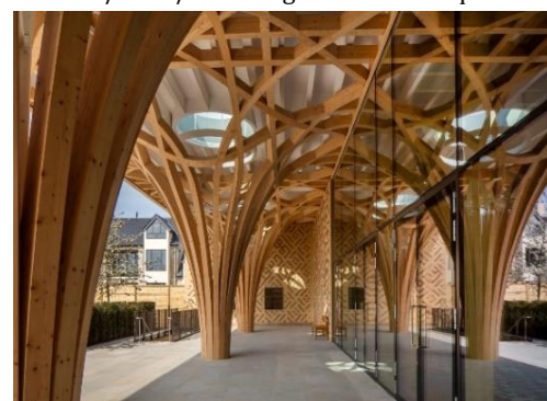
Figure 11. Marks Barfield Architects used cross-laminated timber as the main material. Source: https://www.dezeen.com/2021/01/20/cambridge-central-mosque-marks-barfield-architects/
