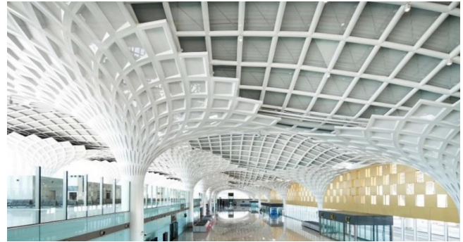
Figure 24. Main Hall: Structure Connection with the Roof Aluminum panels & Level Slab
