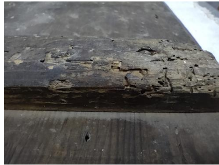
Figure 13. Flight holes and the loss of some wooden parts in the horizontal crossbeams
