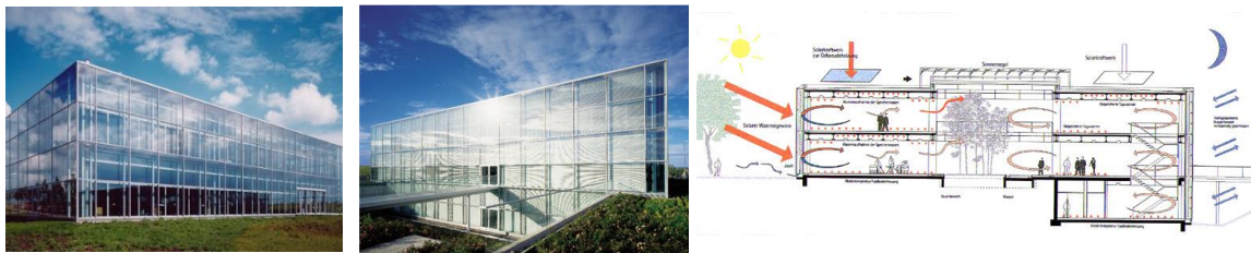
Image No. (3) The GOTZ Headquarters in Germany, designed by Webler Geisser, is a smart, responsive building capable of responding to changes in the internal and external environment, using (BMS), neural networks, and responsive artificial lighting. (17)
