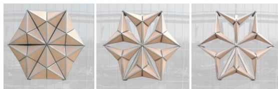
Image No. (12) the movement of the movable shading units of the building. Its design adopts the idea of the mashrabiya, which opens and closes its openings automatically. (15)
