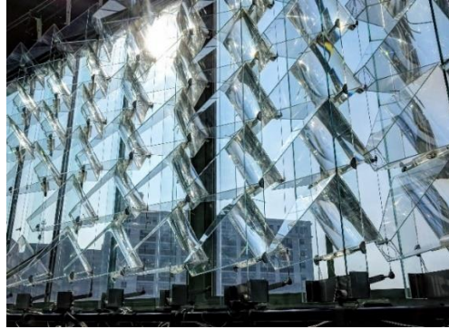
Fig.14: Integrated Concentrating Solar Façade (ICSF)
