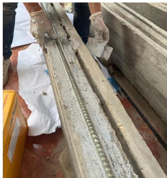
Figure 9. N.S.M F.R.P strengthening technique [63]
