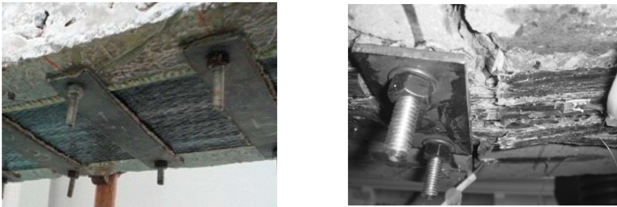
Figure 8. Flexural strengthening using H.F.B-F.R.P [139].
