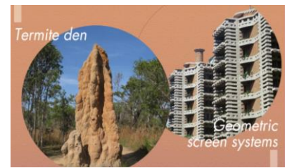
(c). Temperature regulation in the Eastgate Centre office building in Harare, Zimbabwe, inspired by termite mounds.
