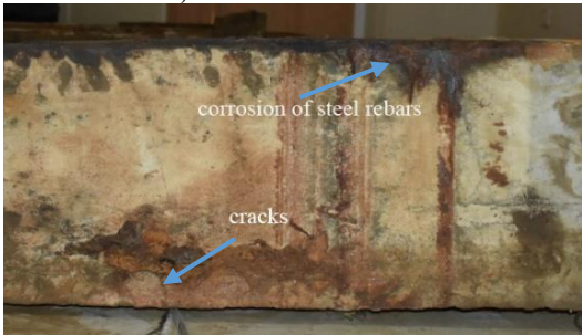
b) Corroded beam
