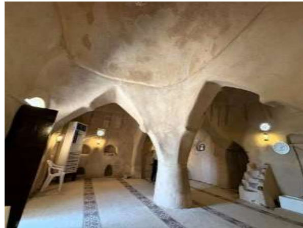
Fig. 15. Al-Bidyah Mosque, the interior of the prayer hall, view from the western corner of the entrance wall showing the qibla wall, mihrab, minbar and a part of the roofing
